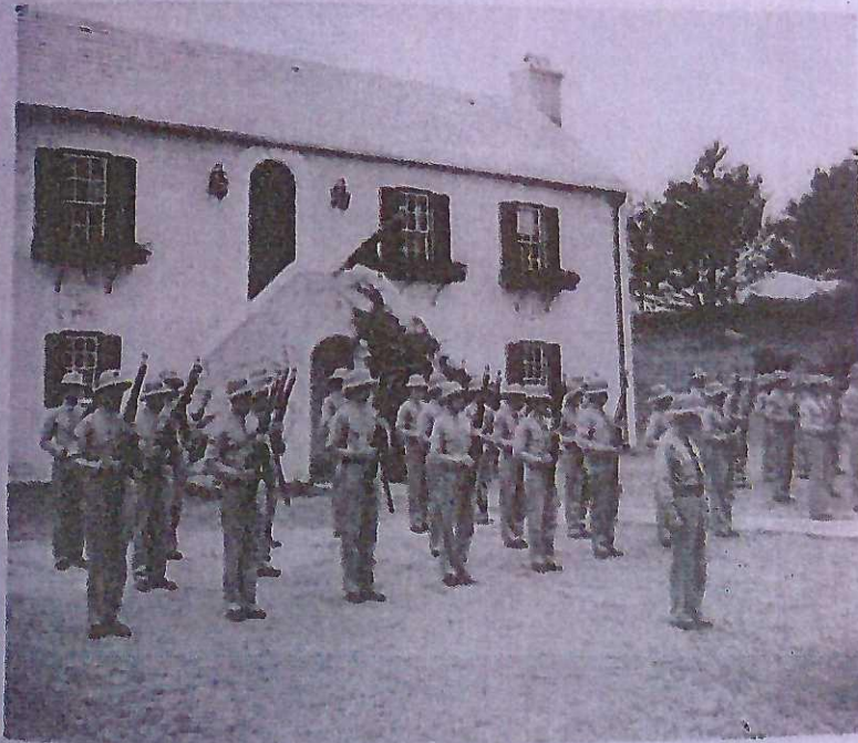
U. S. Marine temporary headquarters is this house on Tucker's Island which was built by Crane plumbing family of Chicago.
